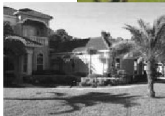
From remodeling a single room to an entire house, the project(s) take time, patience, and expertise. (© Powell Building Contractors, Inc.).
