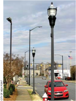
High Point’s LED lighting includes standard and decorative fixtures.
