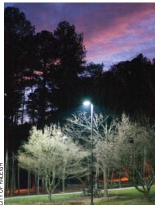
Carolina Pines Park in Raleigh upgraded its parking lot lighting to energy-efficient LED technology.
