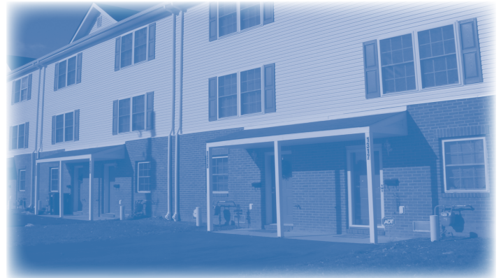
Picture of Greenbridge I, completed
