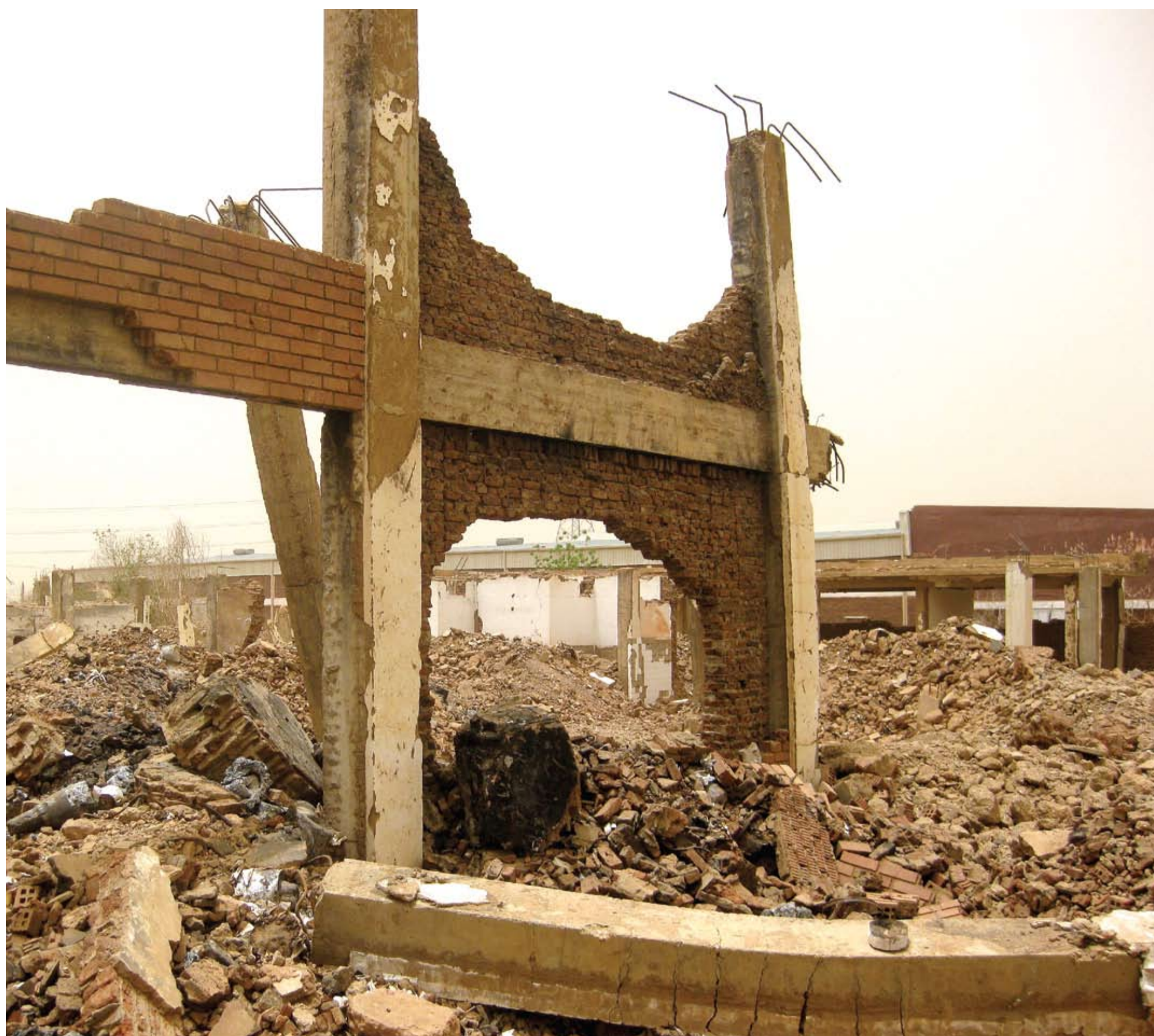
The ruins of the Al Shifa plant which was demolished by 13 Tomahawk cruise missiles launched from a US Navy destroyer. — KT Photos by Conor Purcell
