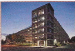
California State University, Sacramento "Parking Structure III"
