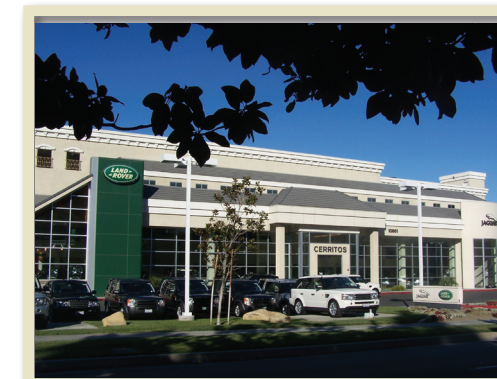
Our State-of-the-art Cerritos Facility
